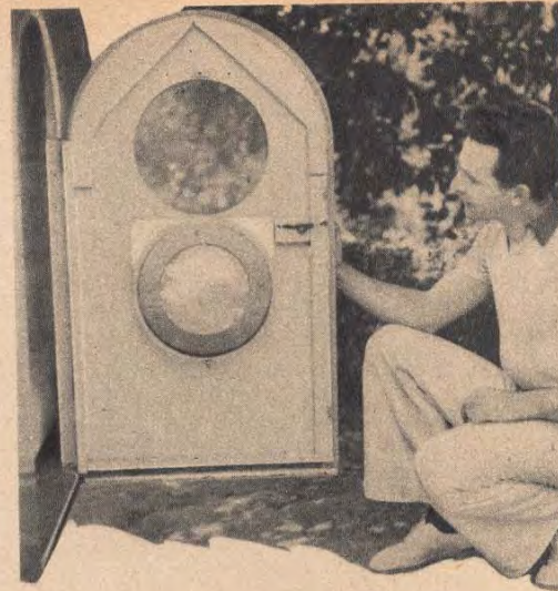
Here is an exceptionally clear picture of the simple door. It may be varied but it is hard to improve for simplicity and sturdy construction. Note the blind door handle box—not shown in the drawings below.
