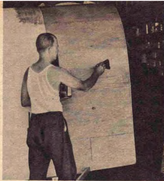
After applying coat of plastic to half of the top, lay on Fiberglass cloth. Pull out all the wrinkles.
