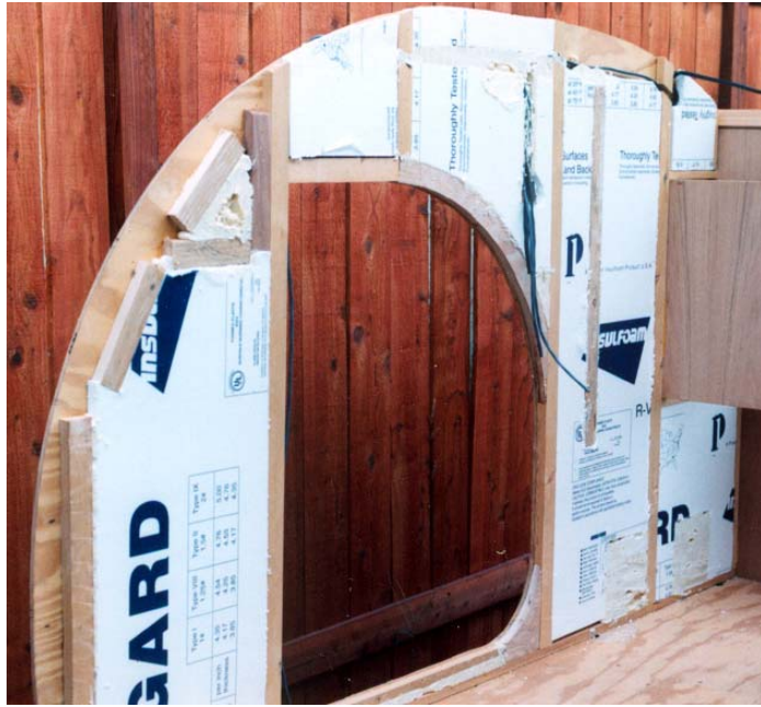
Insulate small spaces with expanding foam. Cut any that expands past the framing with a hacksaw blade. The gaps around the edges are filled after the inside skin is attached.
