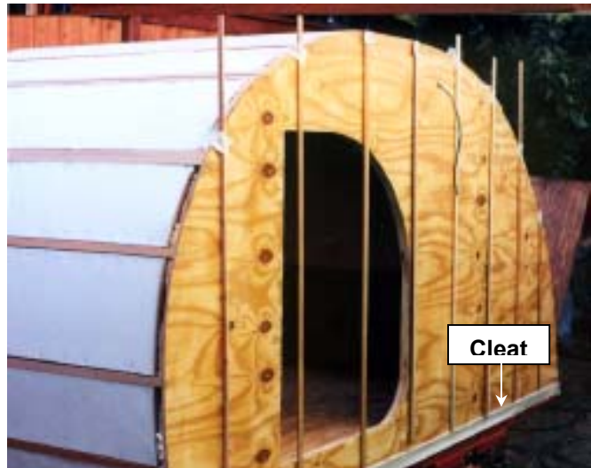
Shims and cleat in place, ready for aluminum.
