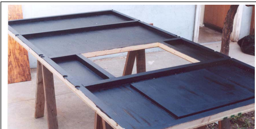
Bottom of deck coated with asphalt emulsion to prevent rot. When this dries, it would be an excellent time to insulate.
