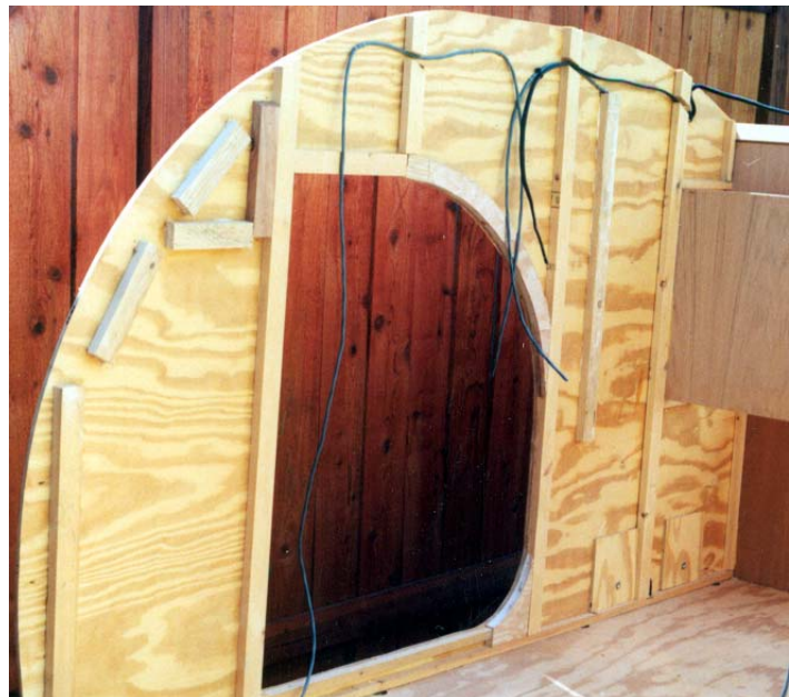
Framing is notched for wiring to pass through.
