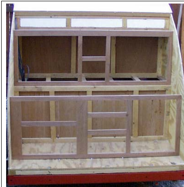
Galley face frames set temporarily in place to correctly position the backing in the shear walls for the drawer guides. (The shop drawings show the correct locations.)
