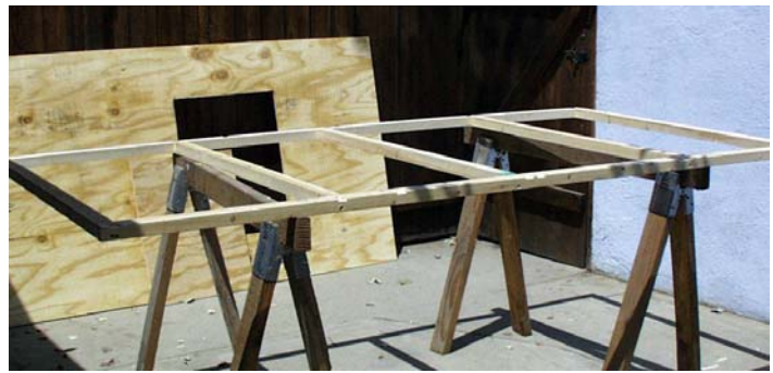
Assembling the wood frame.
