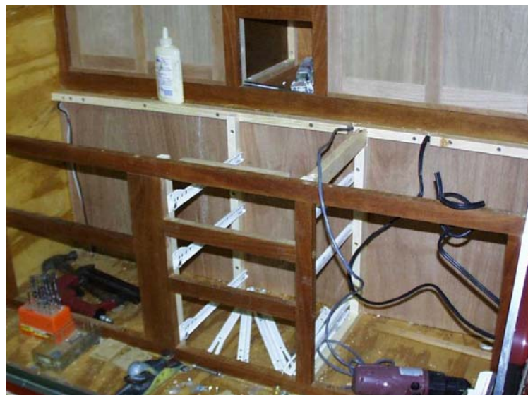
Galley lower cabinet rough-in.
