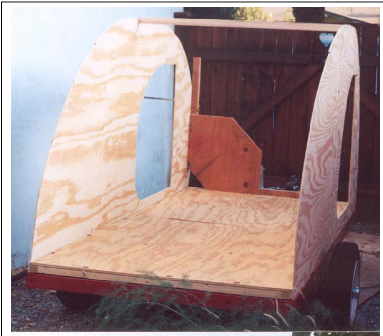
Side assembly. Note temporary spar and right-angle jig.
