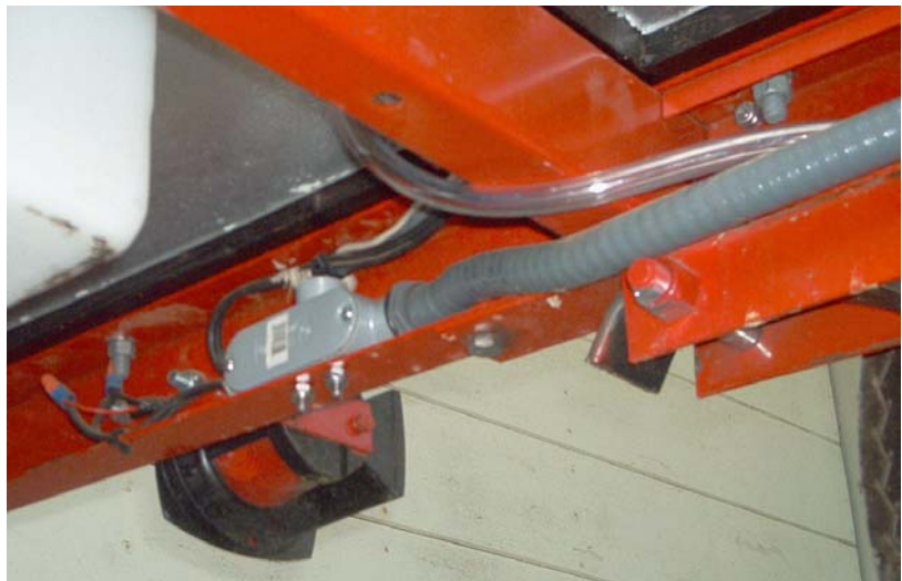
Conduit body at rear of trailer where wiring from fuse box and taillights enters. Clear tube is drain from icebox, which normally hangs straight down.
