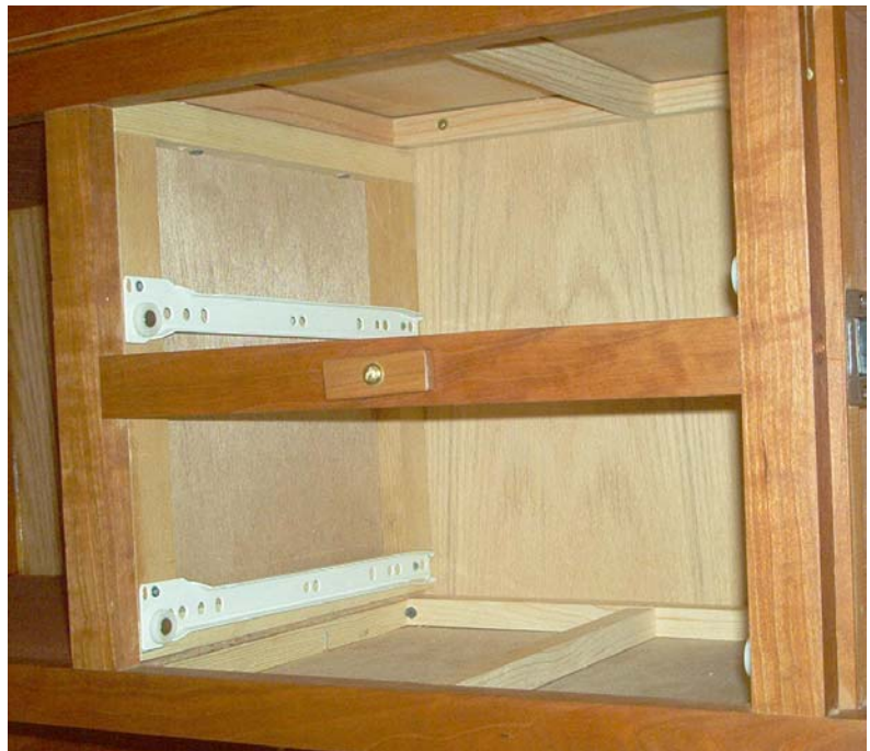
Two shelf support assemblies are visible here: one at the top and one at the bottom. A square roller guide support frame is then screwed into the top and bottom shelf supports, and the roller guides are attached to them. The resulting boxes are then skinned with 1/8" plywood to form the finished cabinet interior. The drawer cavities are left as is.
