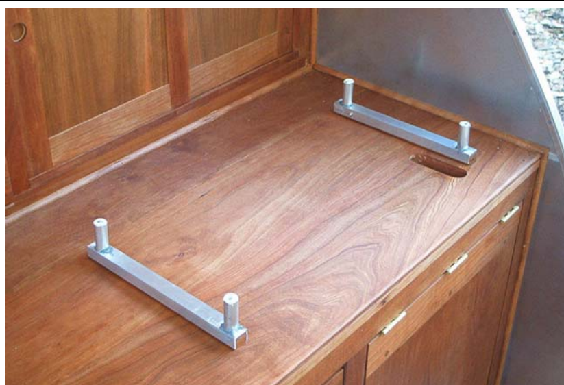
Sliding brackets for stove mounting. The slot at the right is for the LP gas hose. Center the inlet fitting on the stove to move the slot on the countertop farther back out of sight.
