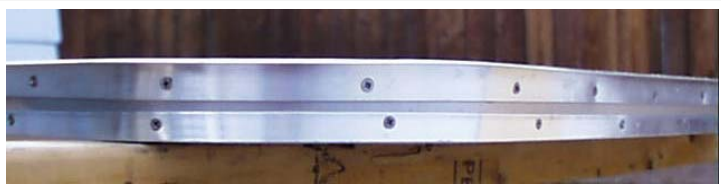
Countersunk screw heads on door radius trim.
