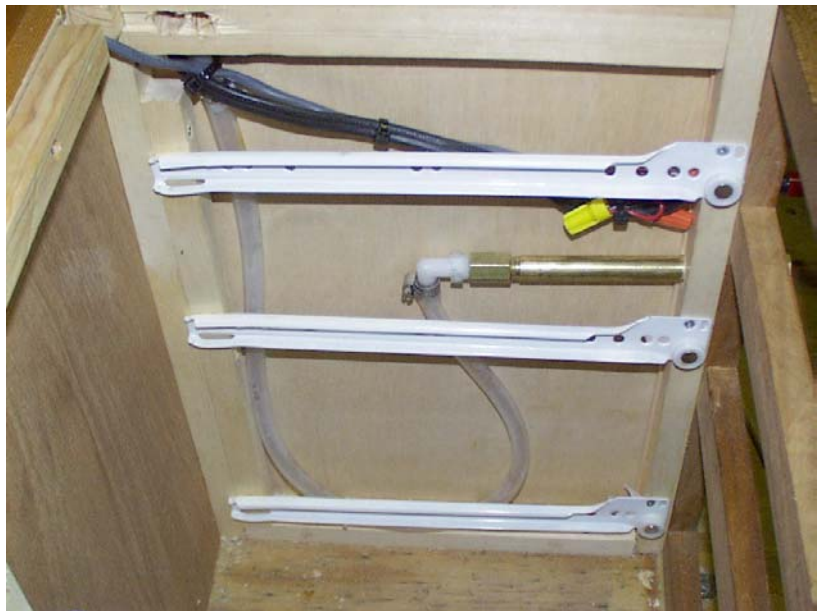
View of the right-hand drawer rollers showing the plumbing for the sliding water spigot and wiring for the pump pushbutton.
