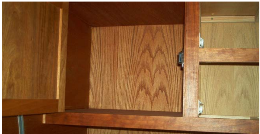
Finished cabinet is skinned and has a door strike.
