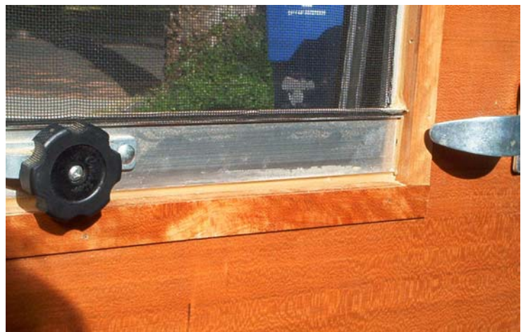
Inside window reveal trim.
