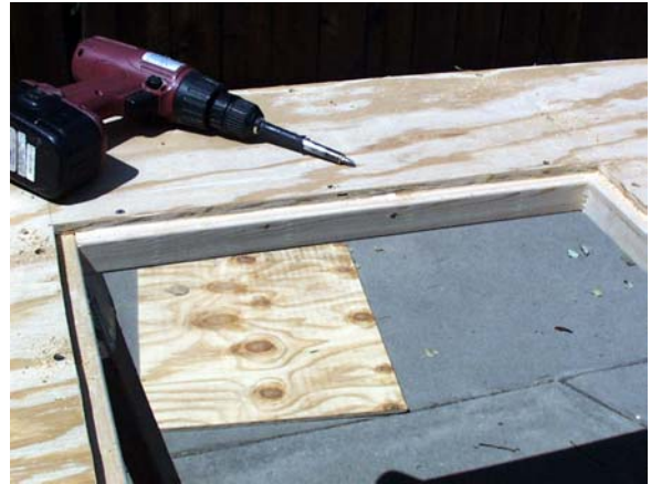
Install the 2x2s on the sides of the hatch opening using glue and screws, centering the 2x2 under the edge of the hatch.
