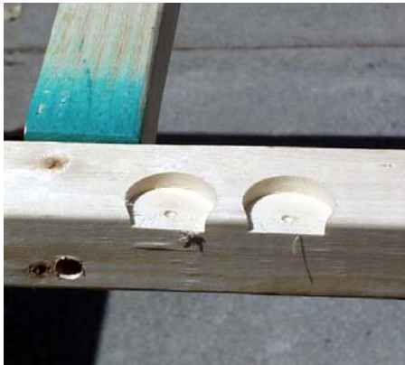
Relief holes where the deck must rest on top of bolt heads.
