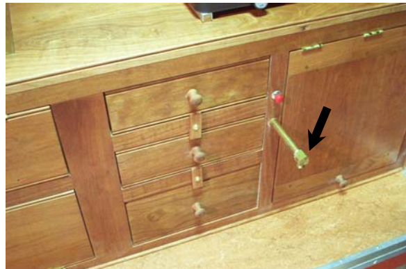
Sliding water spigot in the “closed” and “open” positions.
