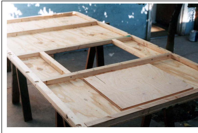
Glue 3/4" plywood under the front of the deck for hanging the spare tire from. Use plenty of glue, then countersink and screw in place from the other side. Not shown is the plywood at the rear of the deck to bolt the water tank to.
