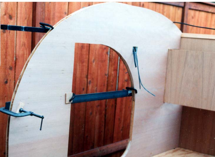
Skinned wall, ready to install spars. Note the angle iron clamped to hold the wall straight.
