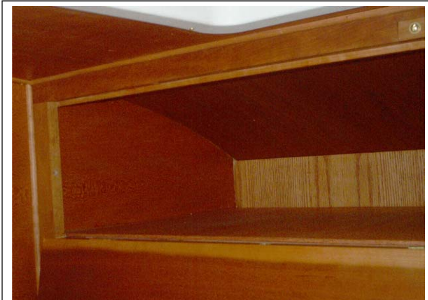
Upper cabinet interior. The bottom is 1/4" plywood.
