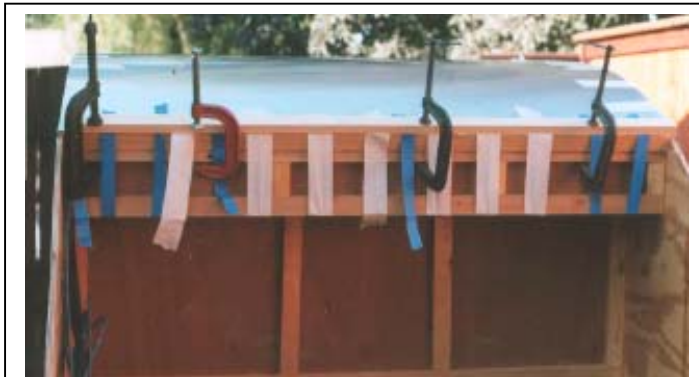
Rear edge of lid temporarily clamped with tape until the cleat is clamped in place with C-clamps. Trim the excess aluminum after the glue dries.
