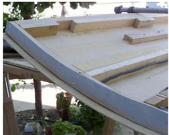
Aluminum edge is pop-riveted onto gusset. Notice the backing for the license plate light and latch.
