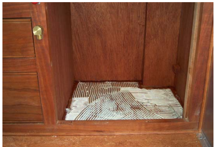
Flooring adhesive. Propane bottle brackets are added after flooring is installed (middle left photo).
