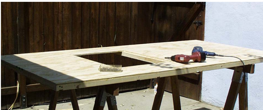
Glue and screw the plywood to the frame. Note the floor hatch cutout (save the piece you cut out).
