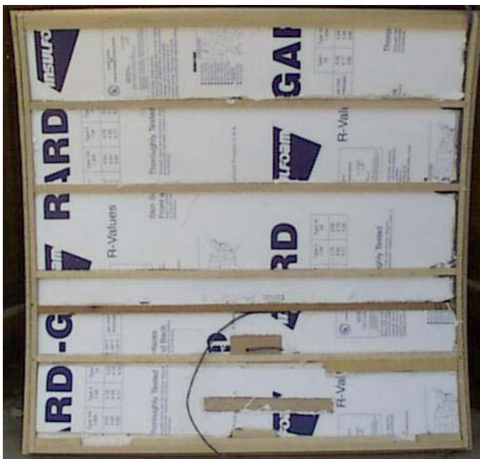
Wired, insulated, and ready for inside skin.
