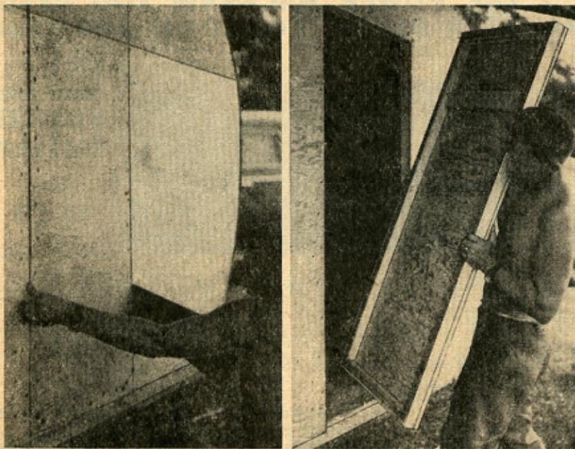
Photo 4 shows the door being sawed out of the sidewall. The door is then lifted out and the edges trimmed. Be sure to leave plenty of play for the metal edge strip, hinges and locks as shown on Photo 5.
