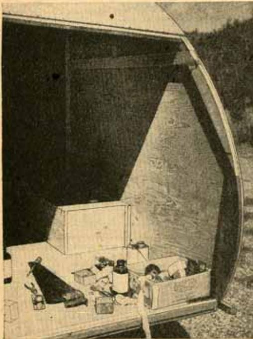
Photo 1. Showing rear end segments glued and screwed to sidewall. Also note splice batten and wheel house box.
