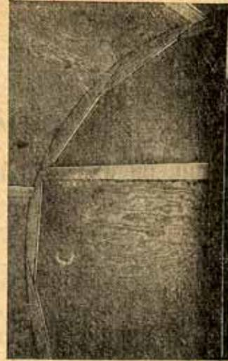
Photo 2. Showing front end curved segments and batten splices on the roof and sides.
