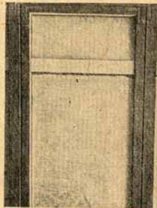
Photo 3. Door jambs and frame are glued and screwed into place first on solid wall.
